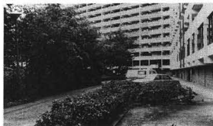
Photo 10. The Bijlmermeer. The "open" courtyard with exotic planting.
