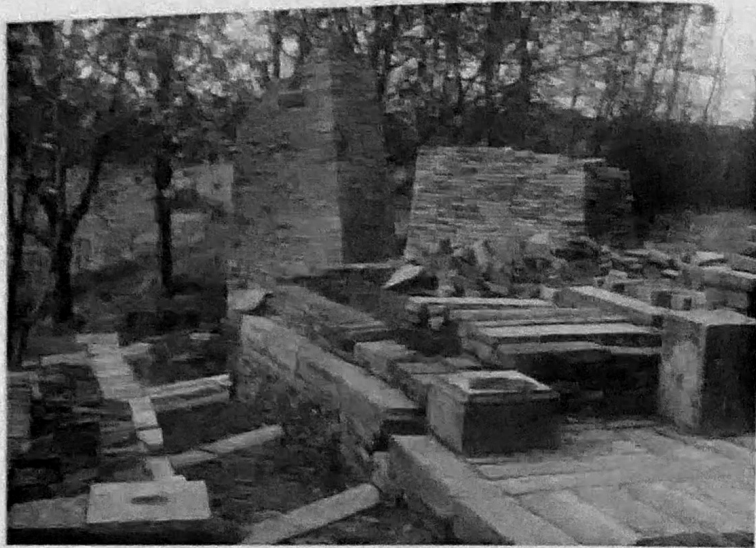
Figure 9 Recycled paving and building materials are stacked in artistic arrangements and form the foundations for Le Roy's eco-cathedral in Mildam.
